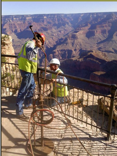
Installing Gordon's railing commission at a Grand Canyon overlook.
